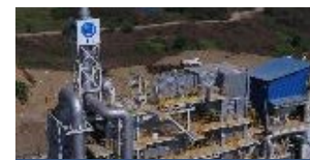
Waste to Energy Plant, JFE engineering, Myanmar
