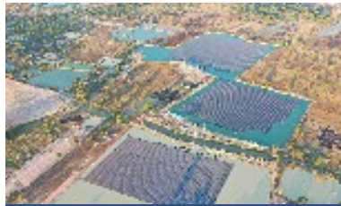
Floating Solar PV, TSB Co., Ltd., Thailand
