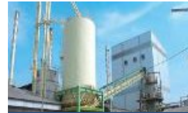
Biomass Co-Generation System, Fuji-Foods Corporation, Thailand
