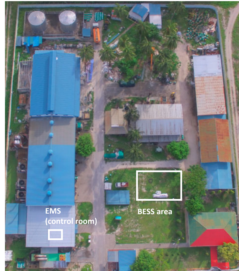
BESS and EMS in Hithadhoo Power station
