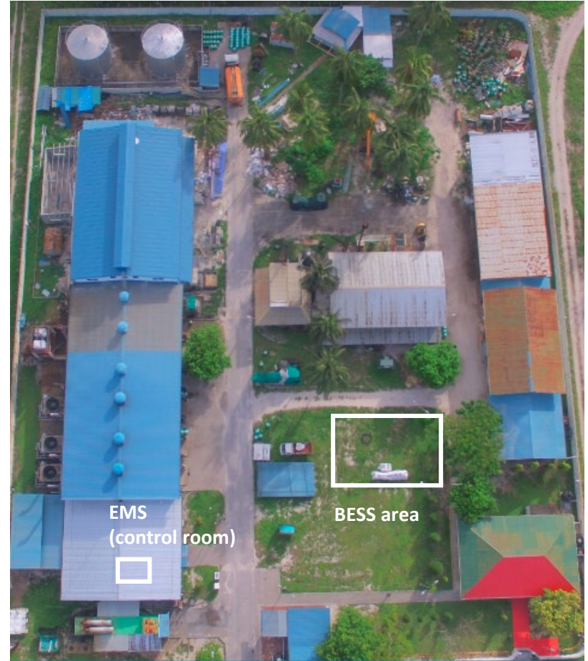
BESS and EMS in Hithadhoo Power station
