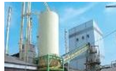
Biomass Co-Generation System, Fuji-Foods Corporation, Thailand
