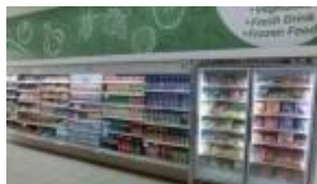
Energy saving at convenience stores, Panasonic, Indonesia
