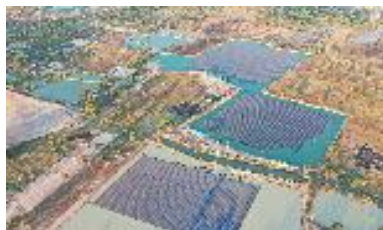
Floating Solar PV, TSB Co., Ltd., Thailand
