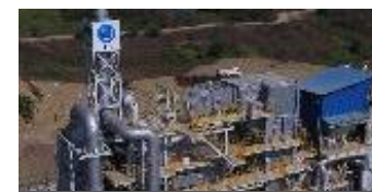
Waste to Energy Plant, JFE engineering, Myanmar
