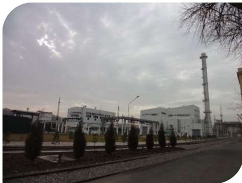
Tashkent Thermal Power Cogeneration Plant
