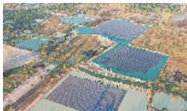
Floating Solar PV, TSB Co., Ltd., Thailand
