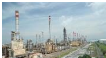
Optimization in petroleum refining plant, Yokogawa Electric Corp. Indonesia
