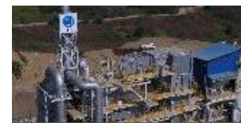
Waste to Energy Plant, JFE engineering, Myanmar
