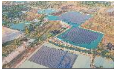
Floating Solar PV, TSB Co., Ltd., Thailand
